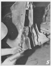
Whe wheel all spot-weld locations, such as the large at the year of the quarter behind the burger and staintess trim. Betind the roof pilot where the quarter window is, there are welds holding the inner quarter to in place; this out the spot welds (Jeff used a Motor Guard weld outter with a built-in diel bit in the center). Fun the drift about 600 rgate, squirling water on it every 15 seconds. This will prolong the life of the cultiers.
