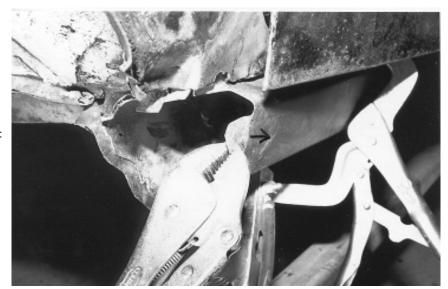
62. Prep the rocker for these braces. Flap it out away from the car toward arrow using vise grips.
